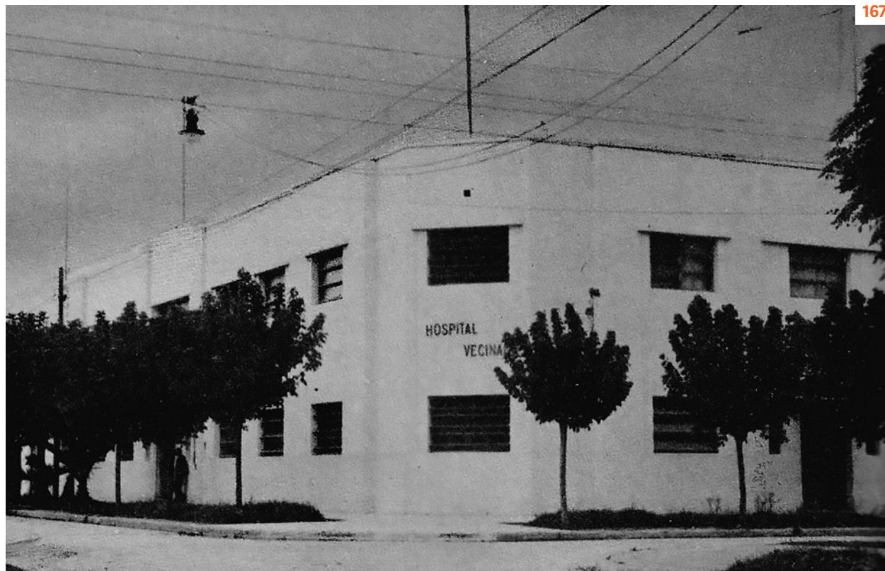
167 Avellaneda Hospital municipal vecinal
